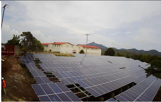
*Photovoltaic solar plant of 289 kW peak, composed of 850 PV modules in Mont-Organisé*
