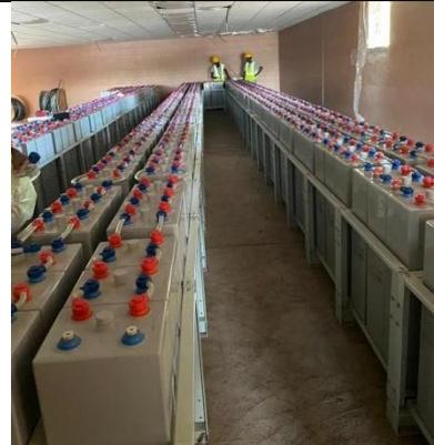
*A bank of 375 storage batteries installed in the technical building of the M-O plant*
